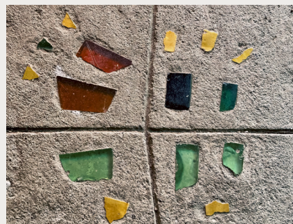
Concrete floor at the entrance with glass inserts
